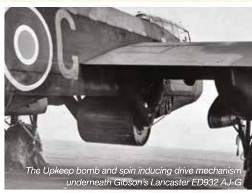
*The Upkeep bomb and spin inducing drive mechanism underneath Gibson’s Lancaster ED932 AJ-G*
